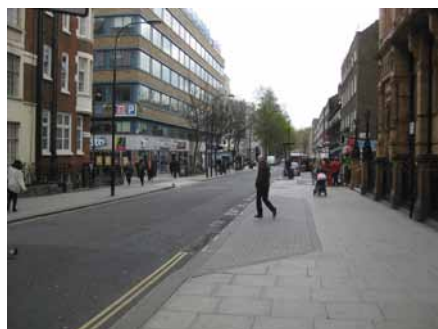
Raised loading bays in Bernard Street
